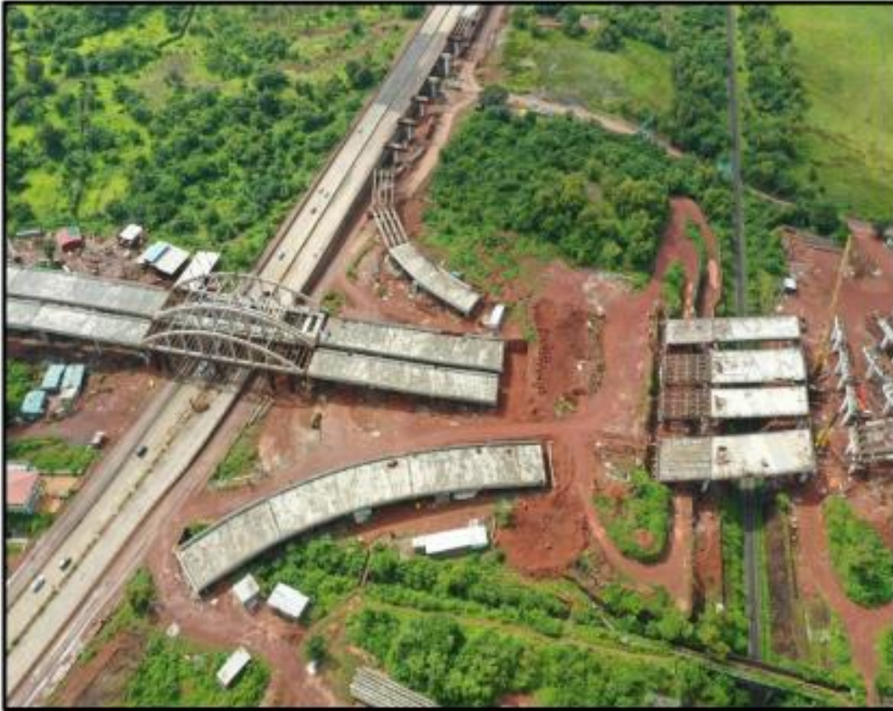
Trumpet Interchange Construction WIP
